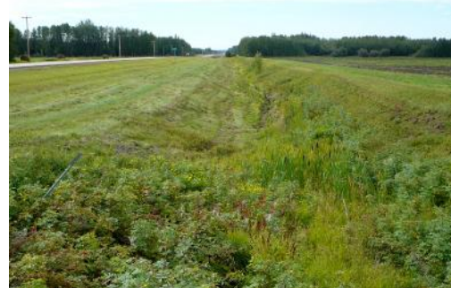
Gordey Drainage Project
