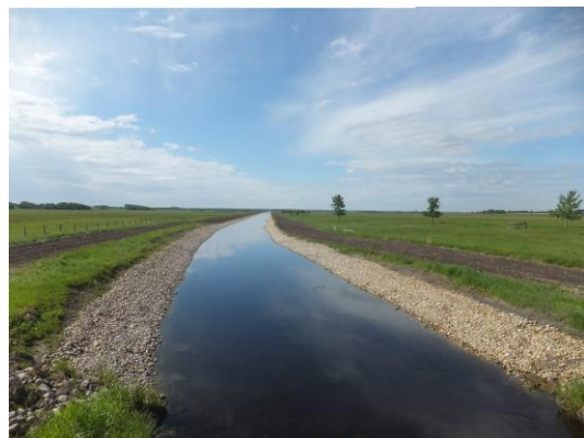
Completed Erosion Control
