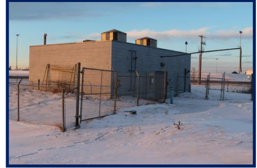
SIP Water Reservoir and Pump House
